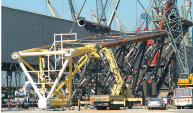
The first gas production tripod is being prepared to move to the job site.
